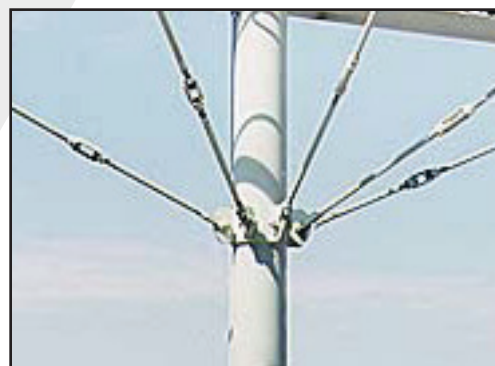
RTA Train Station (Cleveland, Ohio USA)
