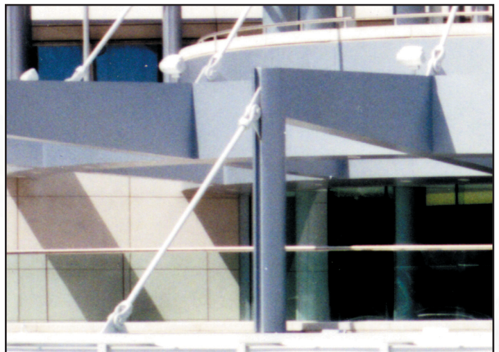
Metro Toronto Convention Centre (Toronto, Ontario Canada)
